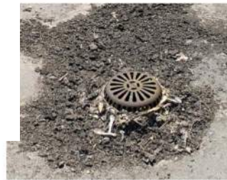
MS, Many drains were severely clogged on the Middle School roofs.
